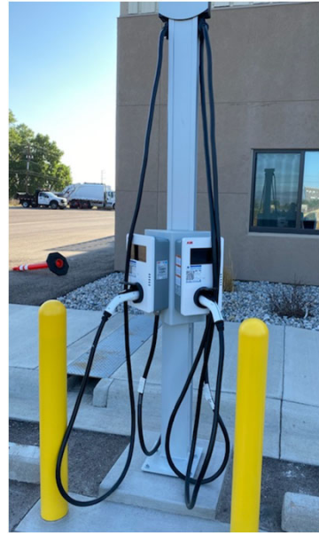
Waste Services (ADA)-South Martin
