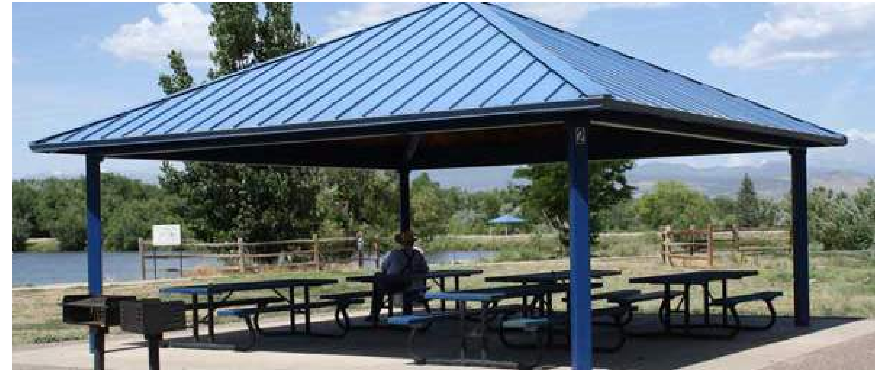
Large Group Picnic Shelter
