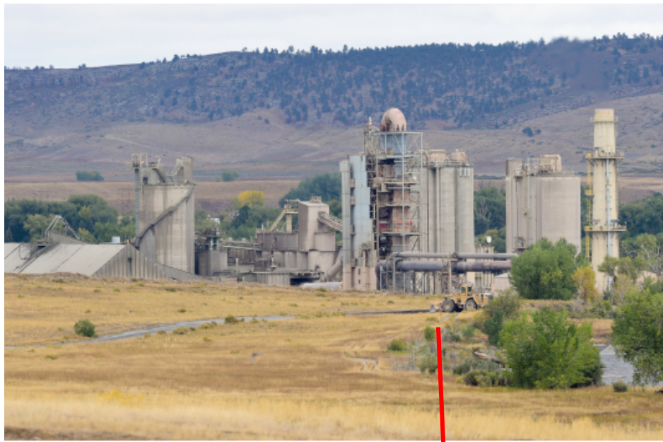
LYONS, CO – OCTOBER 2: The CEMEX Lyons Plant is seen on Oct. 2, 2019. (Photo by Matthew Jonas, Staff Photographer)
