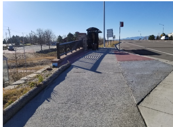
Newly constructed northbound transit stop located south of the Ken Pratt Boulevard and Hover Street intersection.
