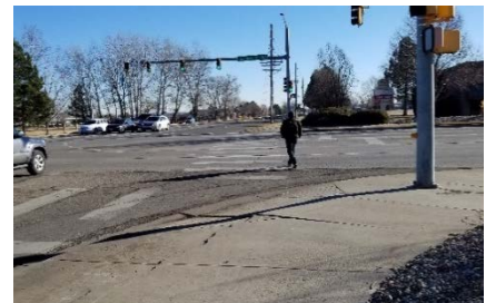
Pedestrian crossing area at Hover Street and Nelson Road intersection.
