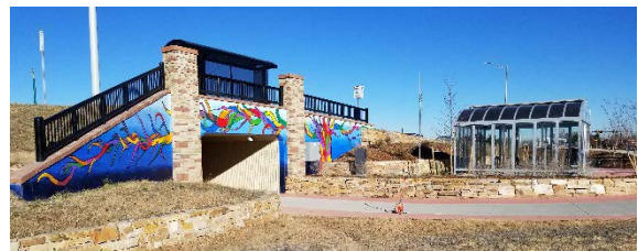
Newly constructed SH 119 underpass west of Hover Street.
