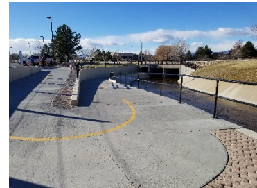
Newly constructed Hover Street underpass south of Bent Way.
