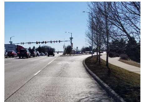
View from southbound right turn lane of pedestrian crossing warning sign at Ken Pratt Boulevard and Hover Street.
