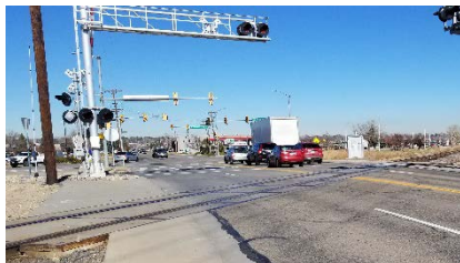
At-grade rail crossing and narrow sidewalks south of skewed Ken Pratt Boulevard and Sunset Street.
