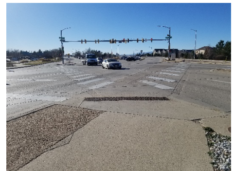
Ken Pratt Boulevard and Hover Street intersection.
