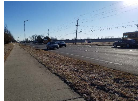
Nelson Road between Hover Street and Sunset Street.
