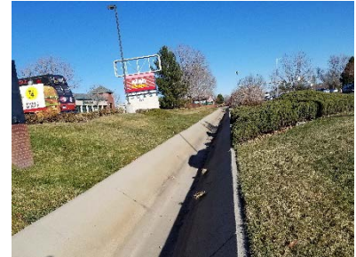
Concrete drainage ditch on west side of Hover Street.
